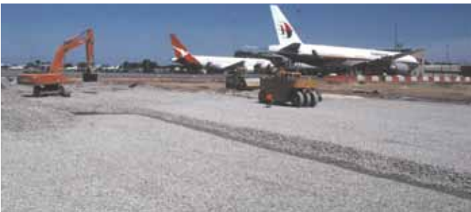
New taxiway at Adelaide Airport (Australia)
