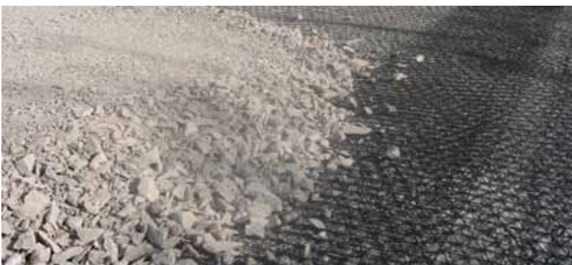
Improving and strengthening the A66 in Melsonby
