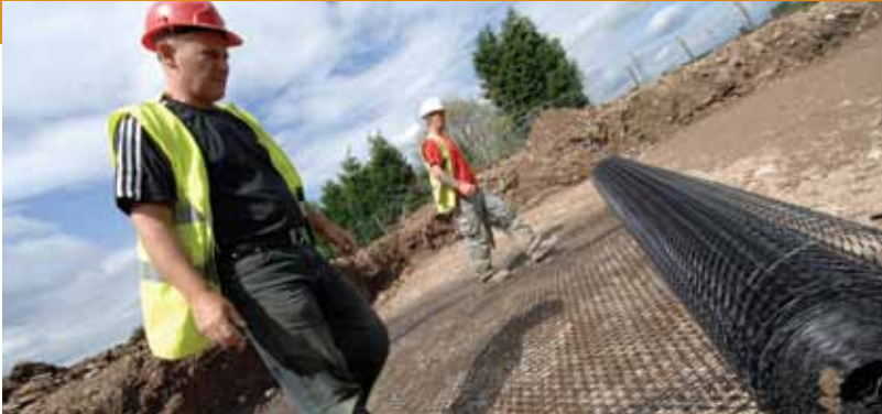
TriAx installation, Stoke
