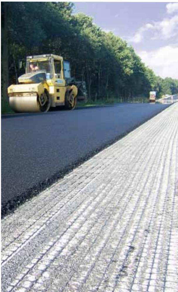
Tensor® AR-G bonds well on to the underlying surface to allow paving directly over the grid.
