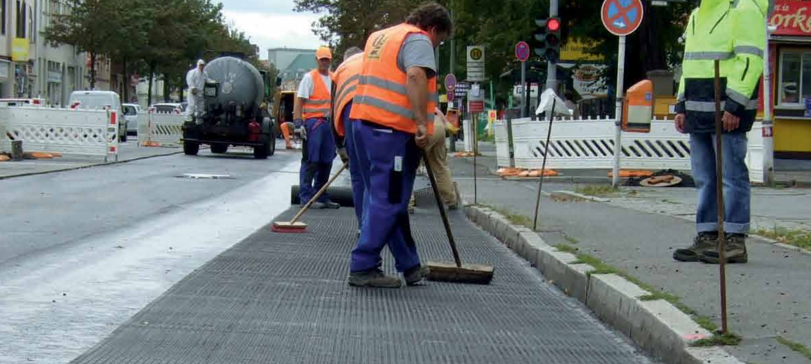
Manual installation of Glasstex®Grid R can be straightforward.
