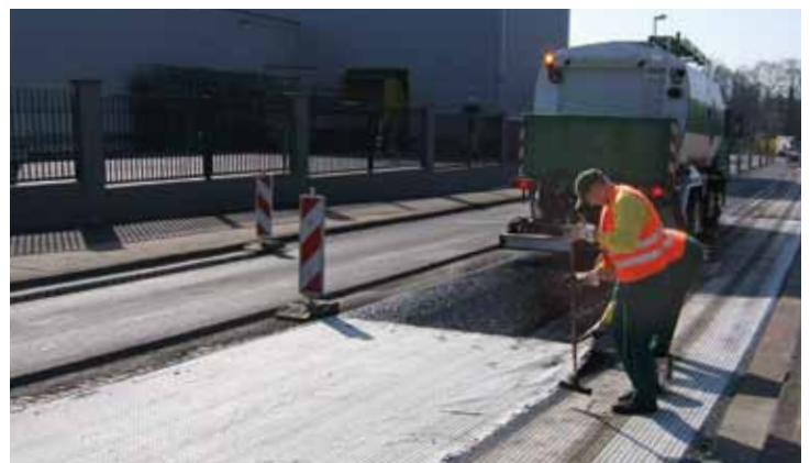
A simple overlap joint for Tensor Glasstex.
