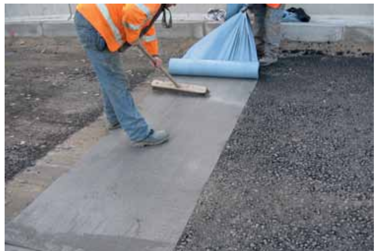
Glasstex®Patch™ 880 can be applied to most sound substrates utilising the adhesive coating.
