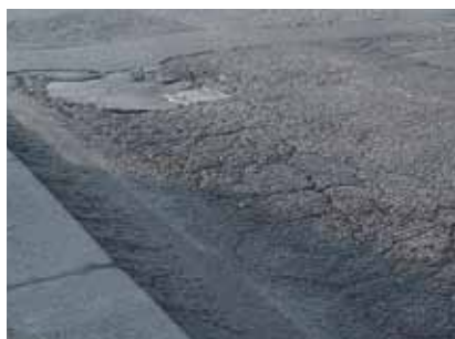
Common structural pavement problems, surface rutting, fatigue and reflective cracking.
