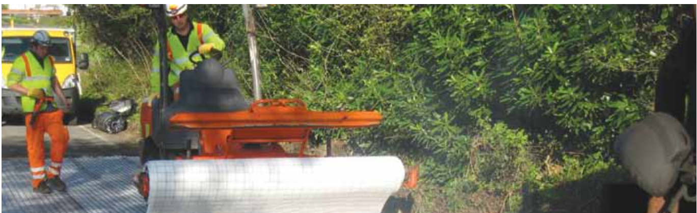
Tensar AR-G can provide resistance to fatigue cracking and minimise fracturing due to long-term differential movements in the subgrade.
