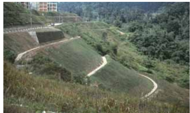
Appropriate face detailing allows vegetation to quickly establish.
