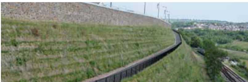
By selecting vegetation to suit local conditions TensarTech GreenSlope soon begins to establish its green face.
