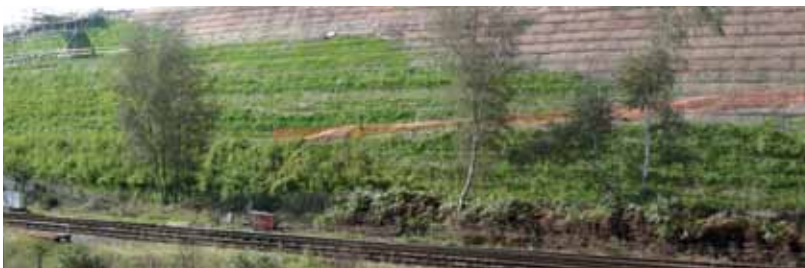
With construction successfully completed, the TensarTech GreenSlope is ready for the vegetation stage.
