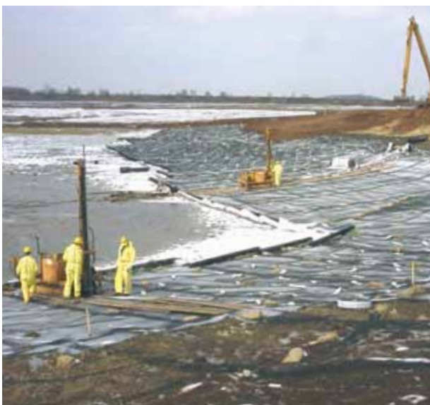
Improved access and a more stable working platform means lagoon capping can be completed quickly and safely.
