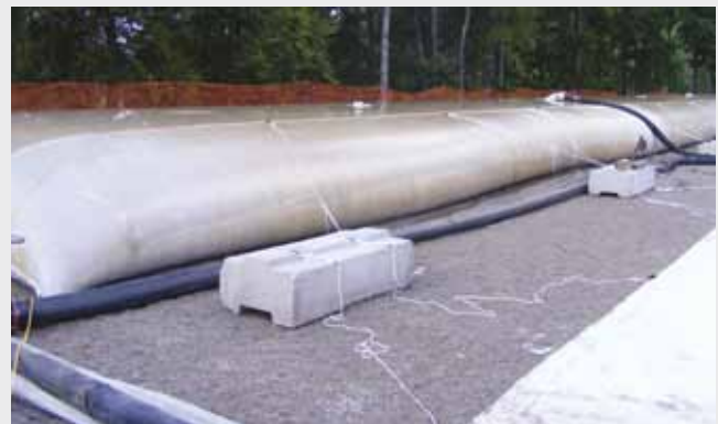
Tensar® Triton geotextile tubes are often cheaper and can outperform other methods in waste dewatering.
