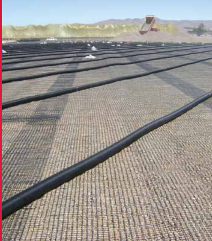
Leach pad construction with Tensar® geogrids.
