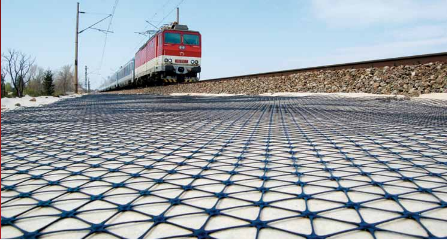
Tensor® geogrid used to stabilise track ballast since the early 1980s.
